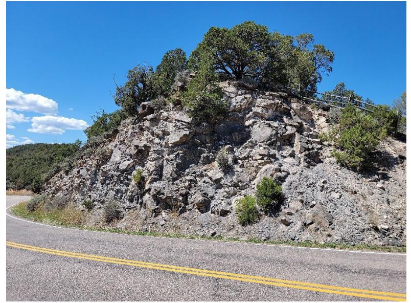
Photo 17. Rock outcrop that will require mitigation
